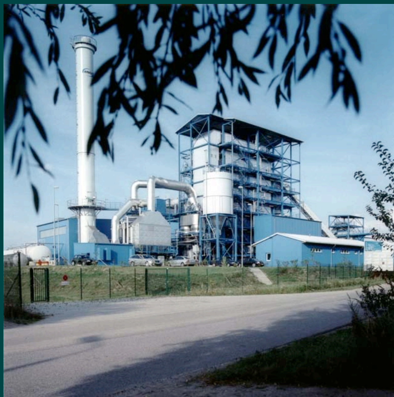
Biomass Power Plant (Siemens)
